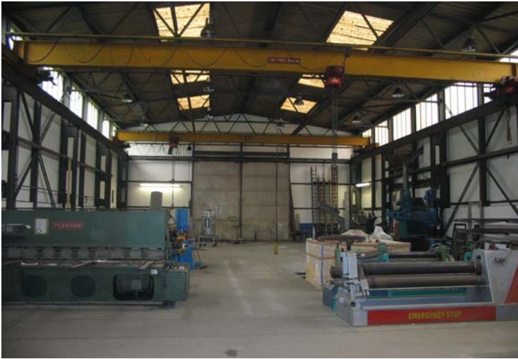
North view of factory hall No 1 (31m x 16m) with overhead cranes
